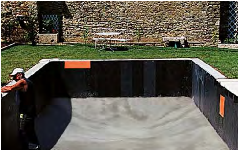
5. SETTING UP COPING STONES
